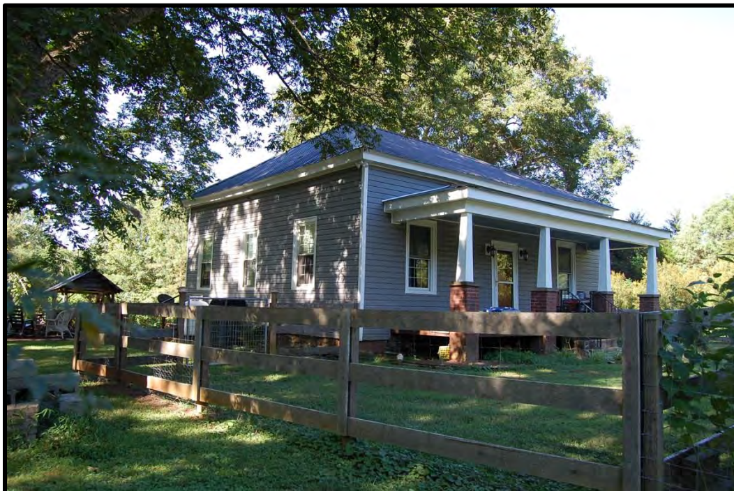
Figure 7. Bobby Bland House, View Southwest.
