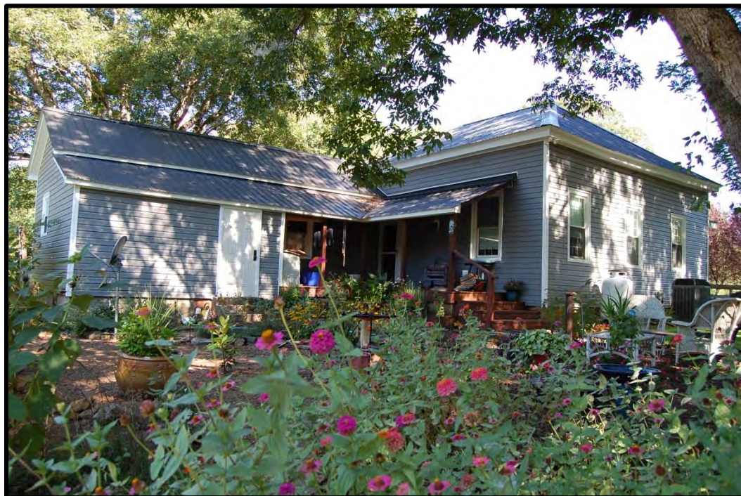
Figure 8. Rear Elevation of Bobby Bland House Showcasing 1920s Addition, View Northwest.
