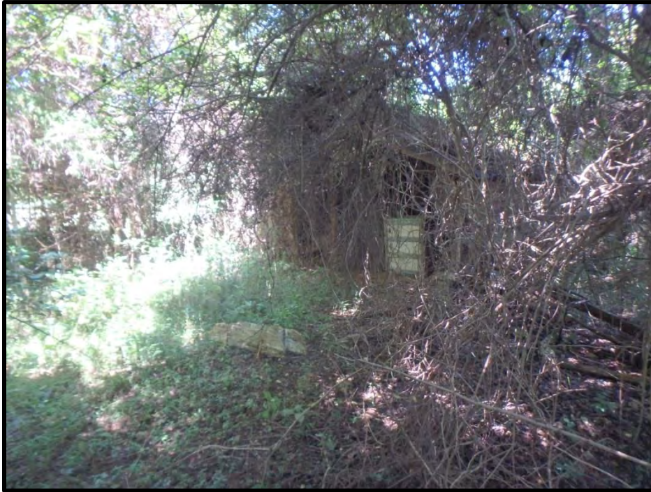
Figure 12. View of Overgrown and Dilapidated Shed in Project Area, View Northwest.
