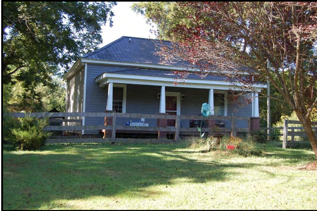
Figure 6. Primary Façade of the Bobby Bland House, View South.
